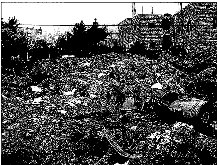
A demolished house in Beit Jala, a Palestinian refugee camp. The house was demolished by the Israeli military to create a "security zone" around the camp. A chair and the hot water tank are still visible in the rubble. Photos by Kate Raphael Bender (see page 7.)
